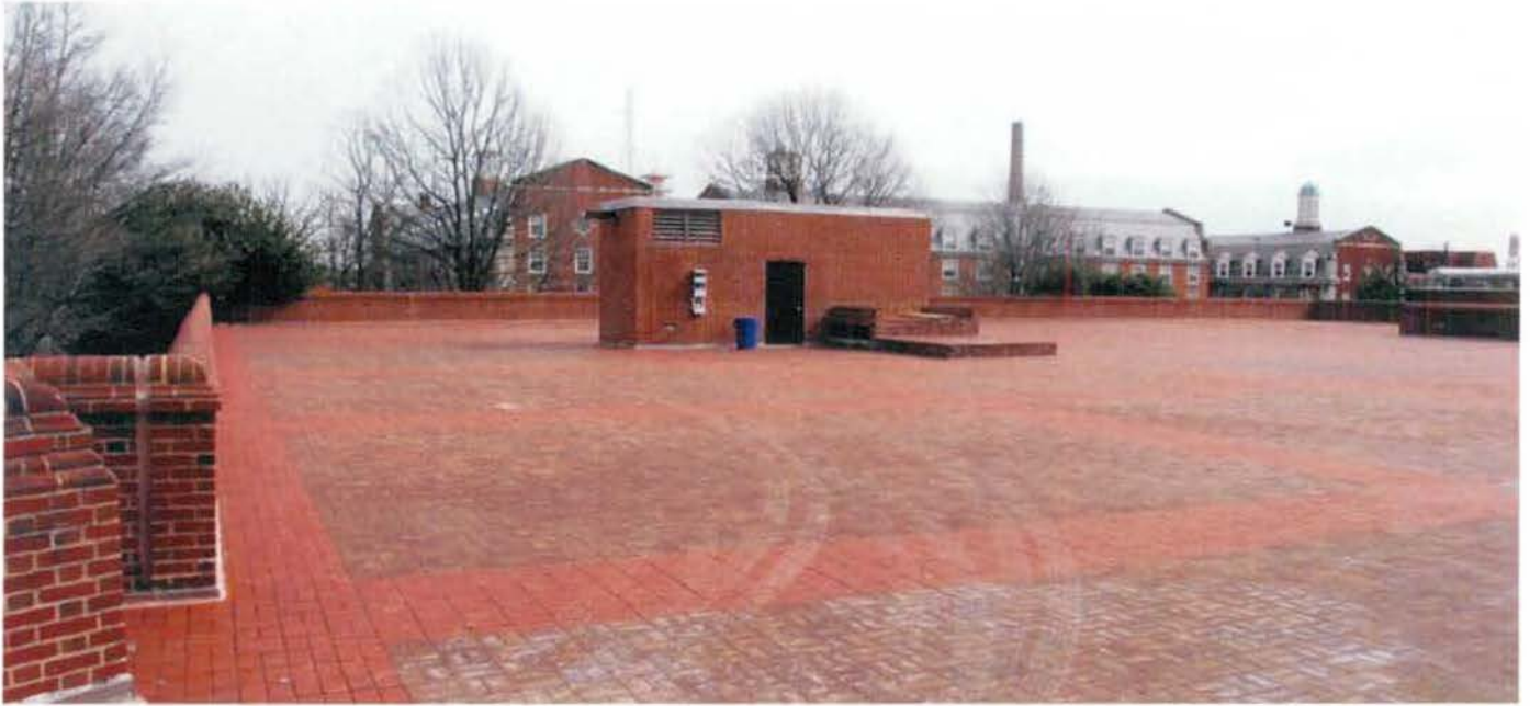
Photo 6-3: View of existing roof of Undergraduate Library
